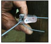
Pull tight against the post and bend the wire under the T-Clip. Cut off excess wire to suit.
