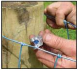
• Wrap the wire around the strainer post and twist the T-Clip onto the line wire.
