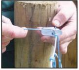
• Push the line wire into the hole in the T-Clip and pull through.
